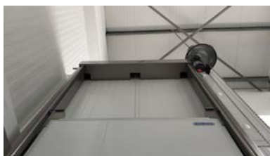
Detail of third safety cable.
