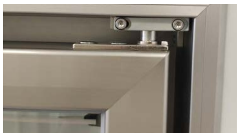
Door top mounting with adjustment
