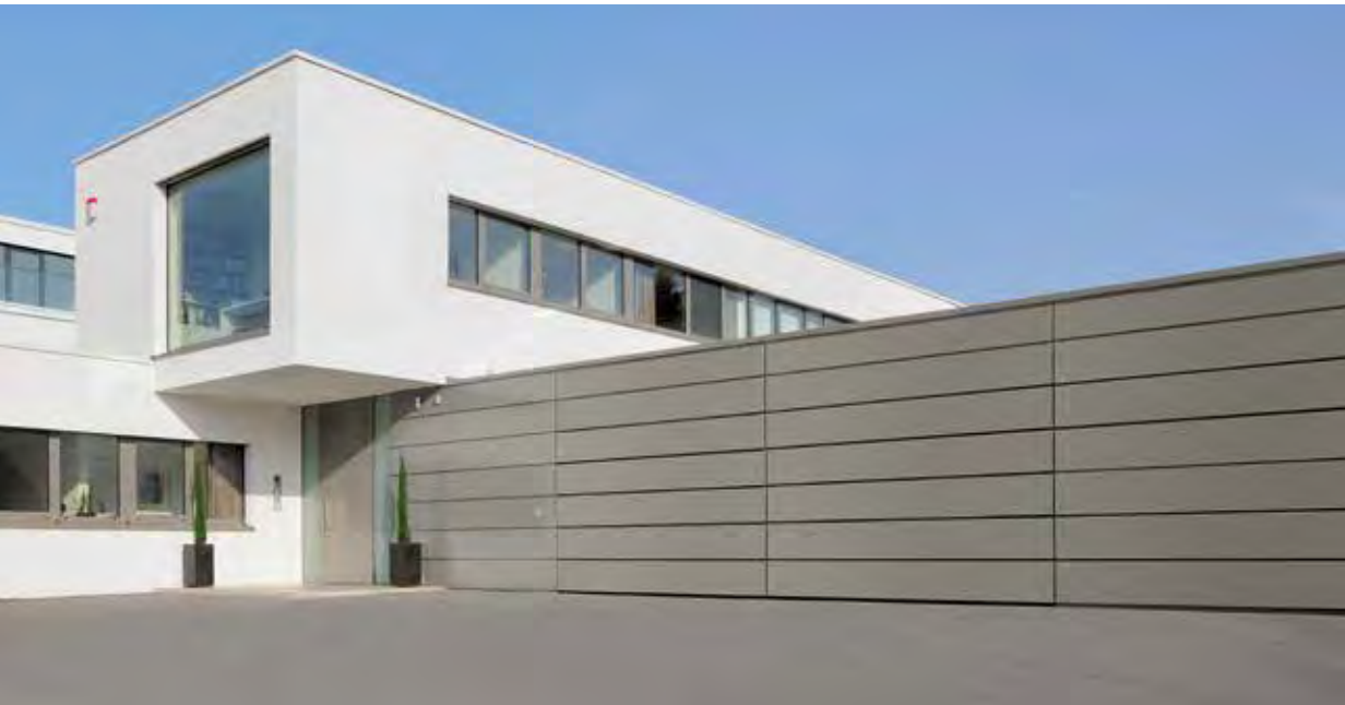
On-site cladding with aluminium compound board
