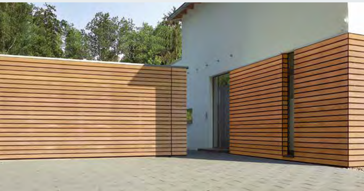
On-site cladding with timber panels
