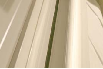
Detail of structure
